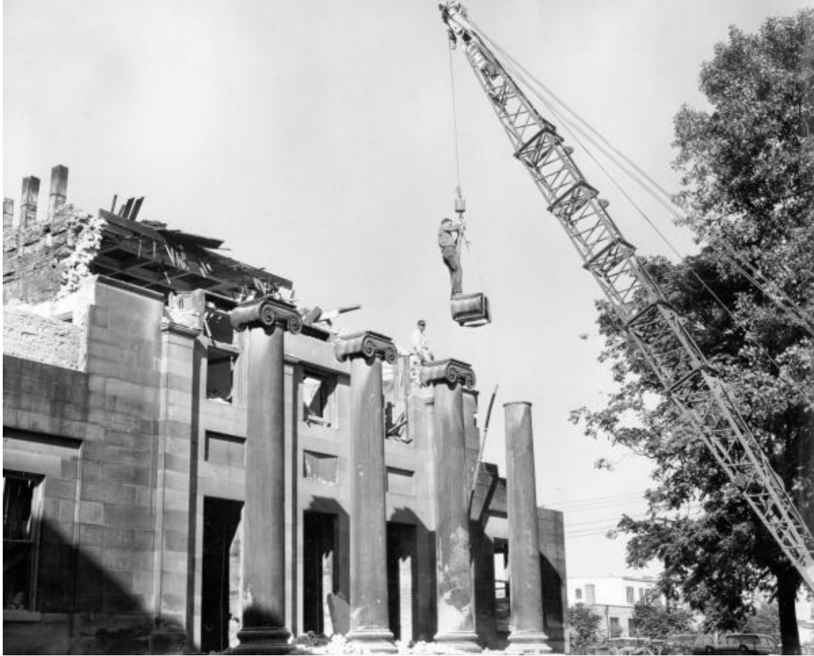
Salvaging the south portico of the Kelley Mansion for relocation, 1961.
